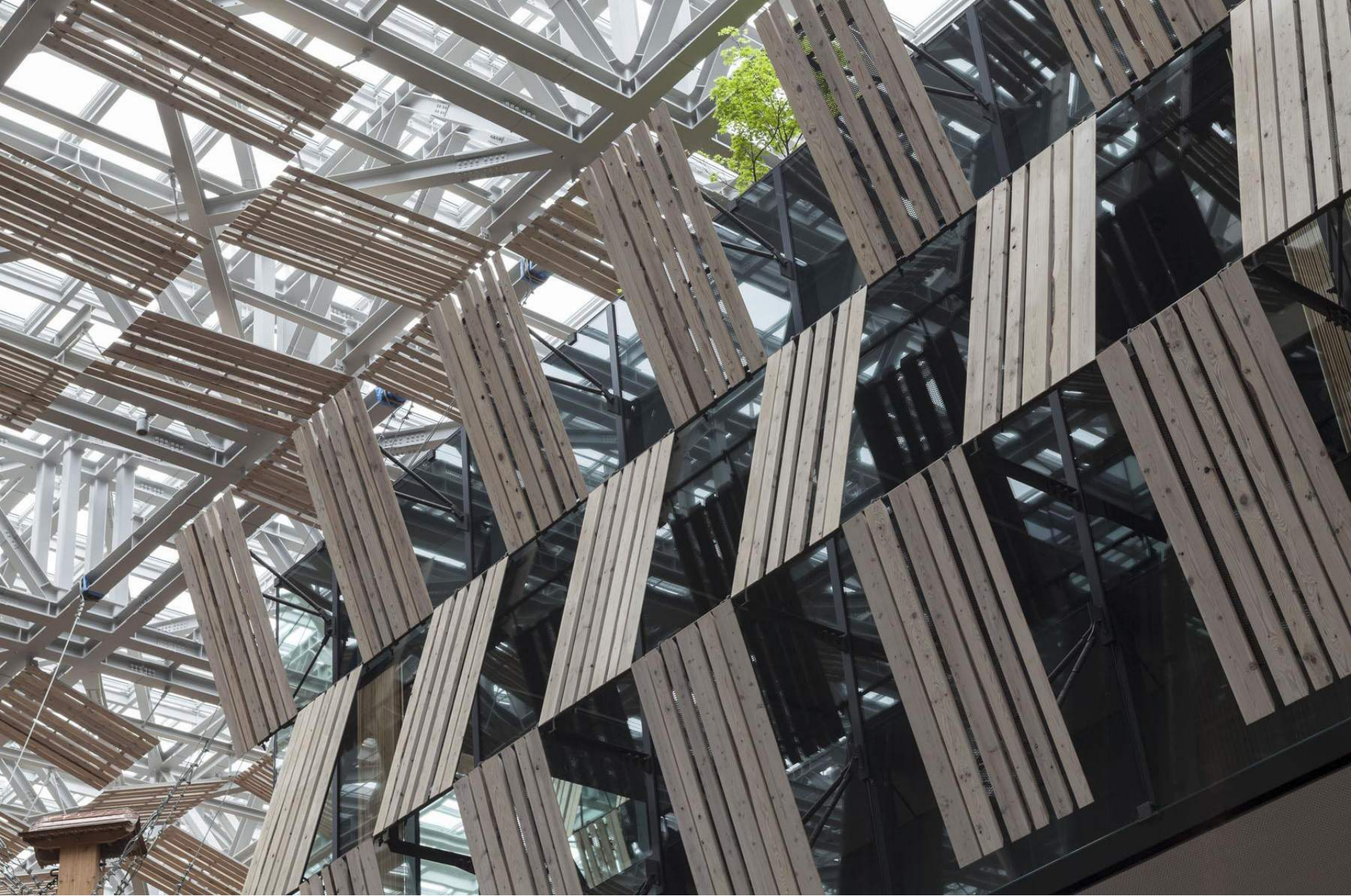
Nagaoka City Hall Aore Project
