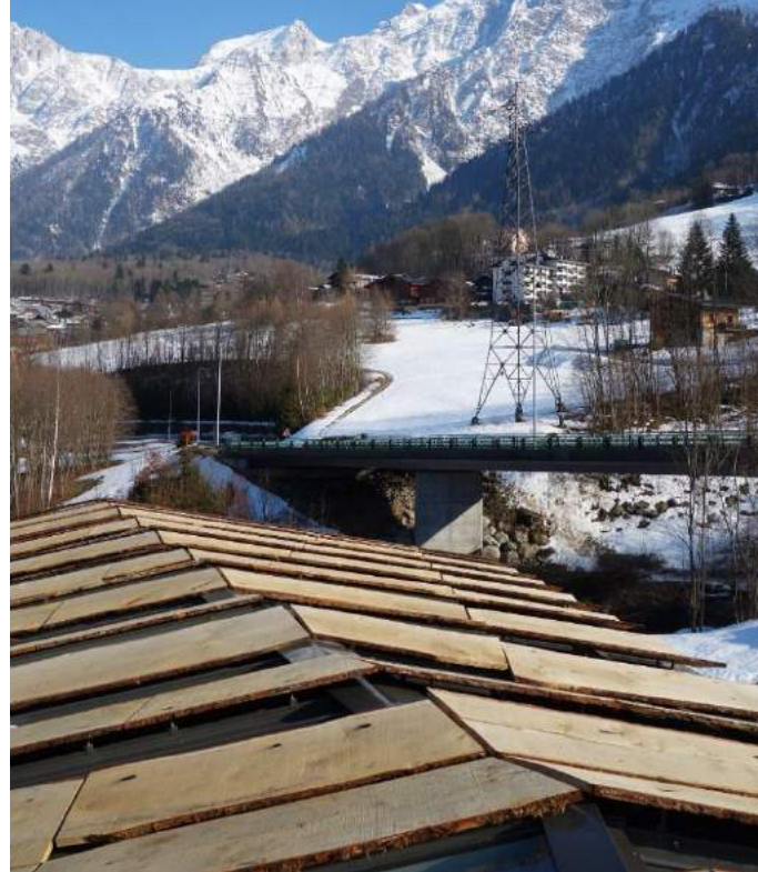
Roof composition : Oak boards – Standing joint aluminum roof - Glass roof
