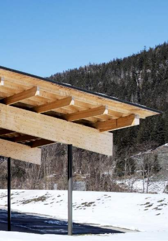
Roof composition : Oak boards – Standing joint aluminum roof - Glass roof
