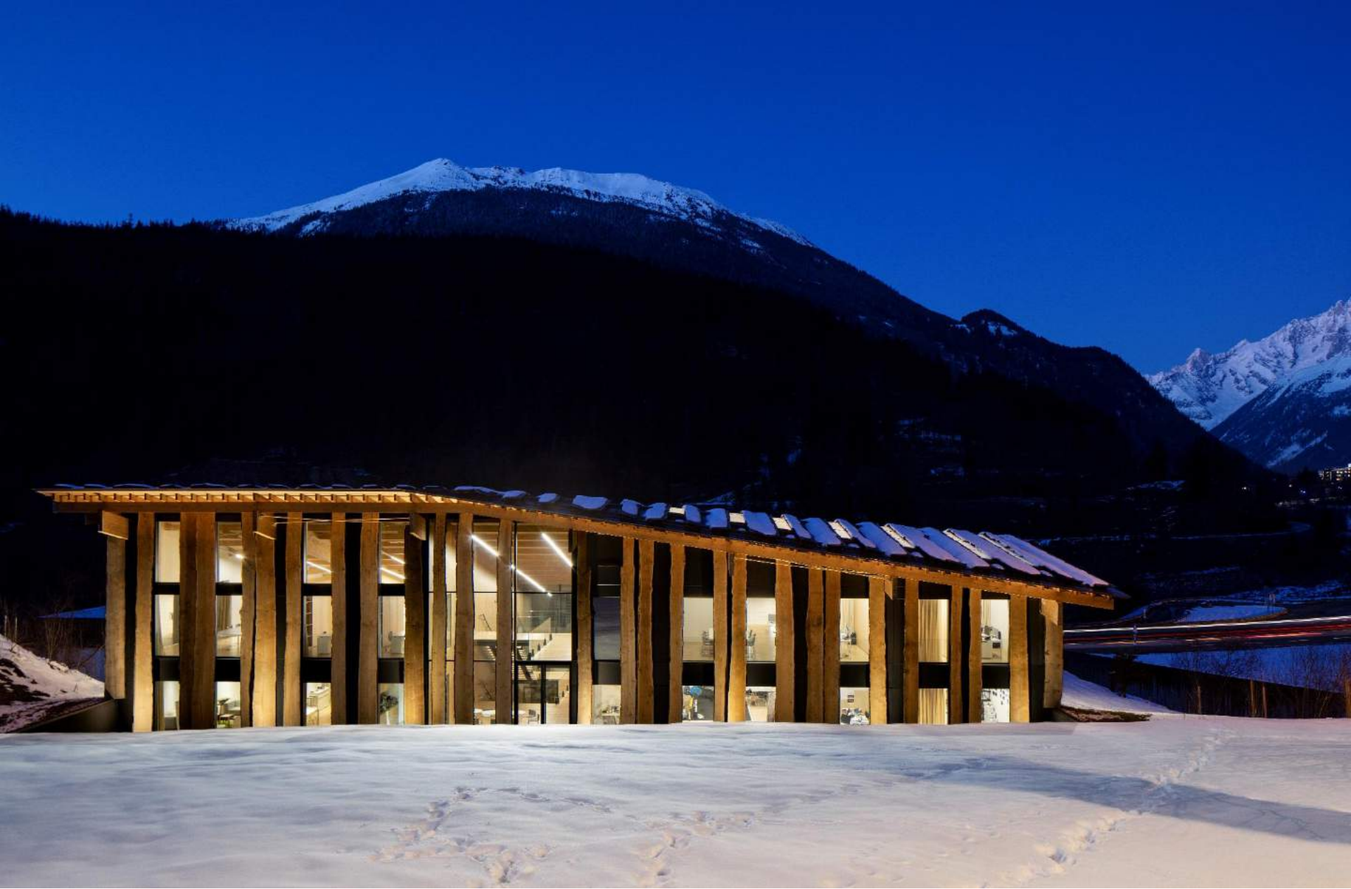
Night view – South Facade
